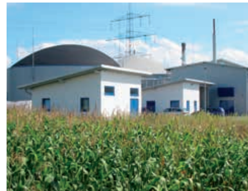
Biomasse-Anlage in Neuried
