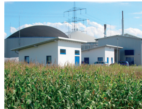
Biomasse-Anlage in Neuried
